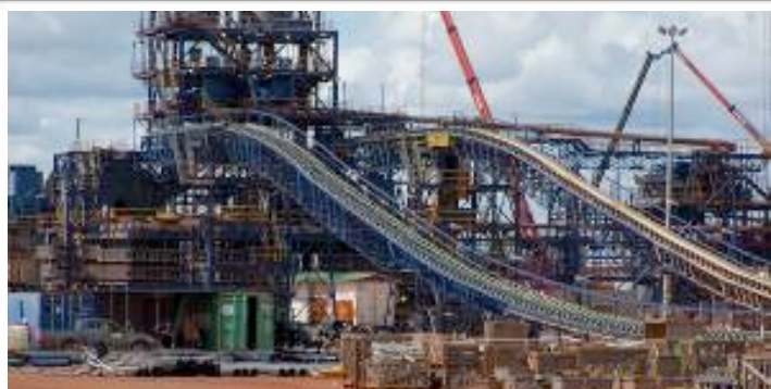
Conveyor Structure and Pipe-racks
