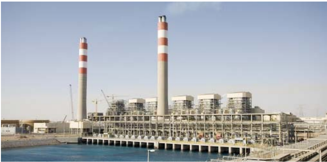
Structural Steel For Shoaiba power plant 5,600 MW
